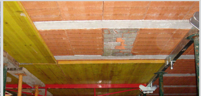
Desencofrado sin reapuntamiento / Decapage sans re-enfort / Un-formwork without props reinforcement
