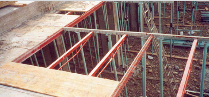
Desencofrado sin reapuntamiento / Decapage sans re-enfort / Un-formwork without props reinforcement
